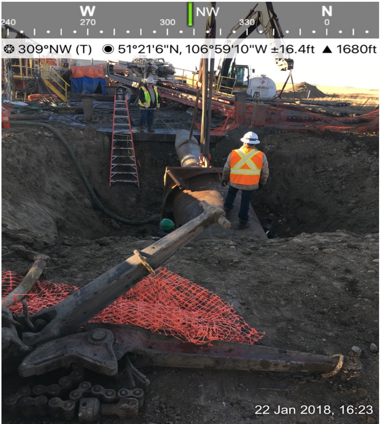
Hammering out the casing
