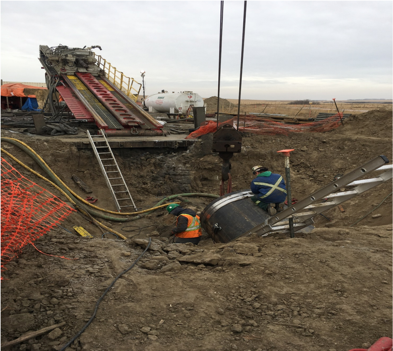
Just finished cutting out some of the casing
