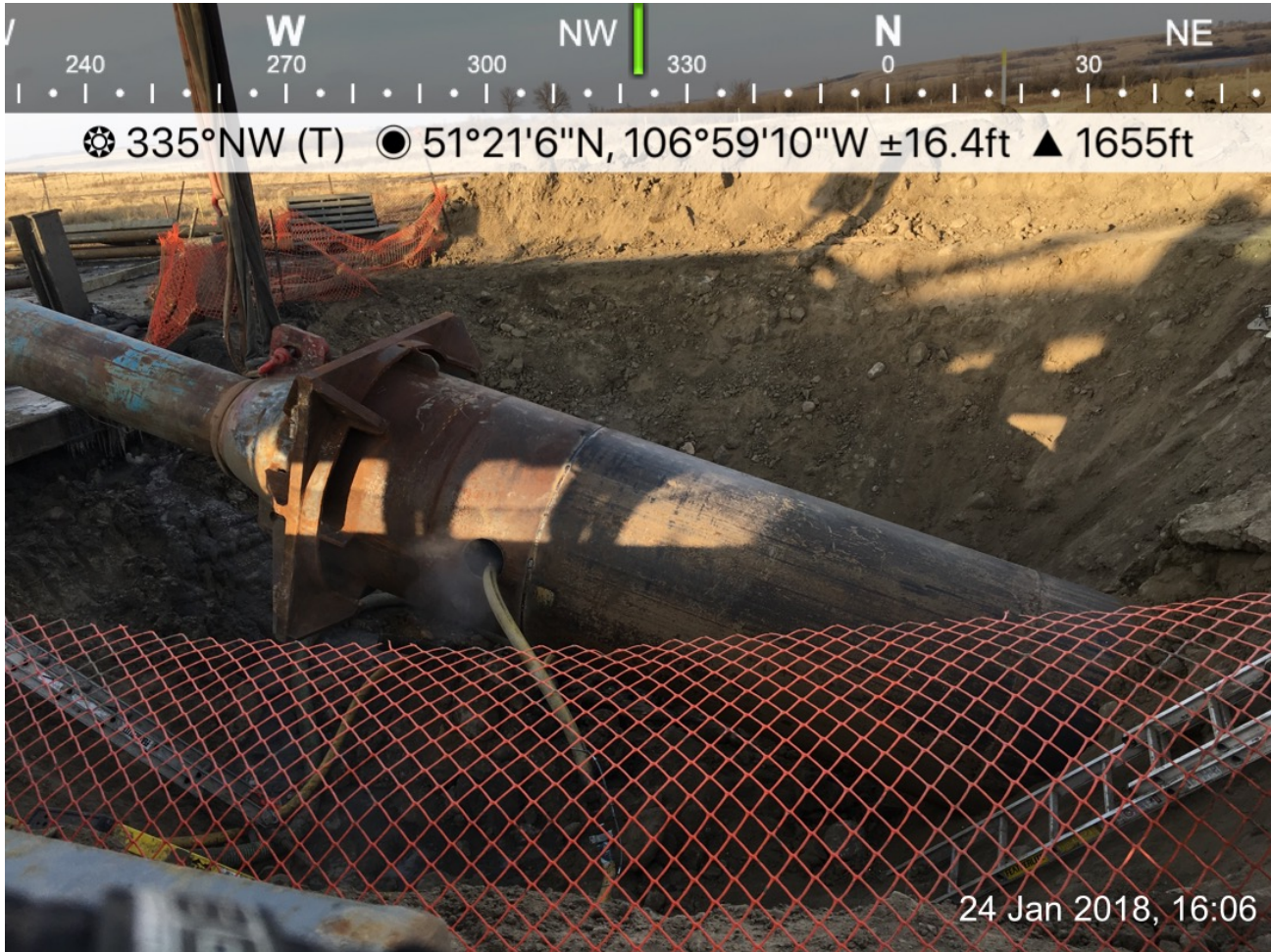
Hammering out the casing
